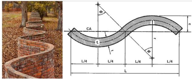
Figure 1: A Crinkle Crankle wall in Suffolk (UK), left. A sketch of the same wall, right.
